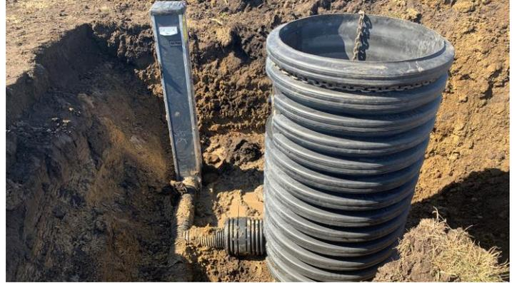
Figure 3. Gate Structures to Control Water Table
